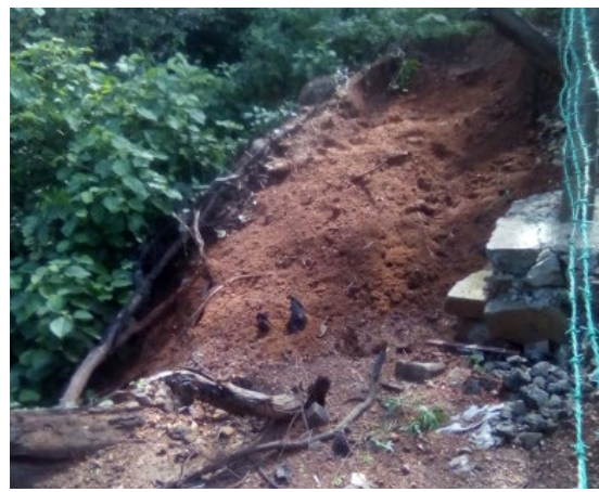
Removed from worksite, 10 Nov. 2021
