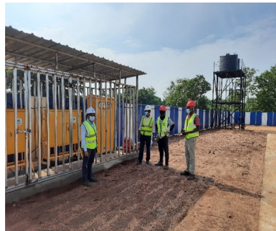
HSE joint site inspection the Engineer the Contractor UEC ICB-2A, 28 Oct. 2021
