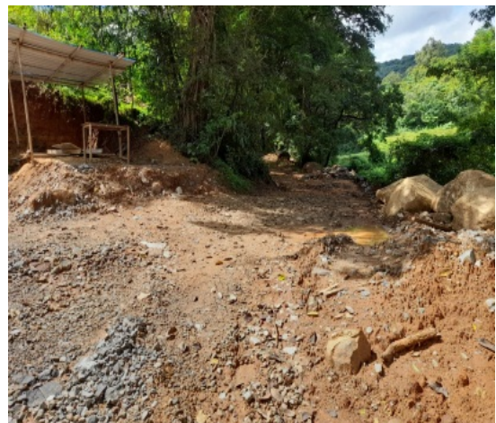
Removed debris from the worksites, 7 Nov. 2021
