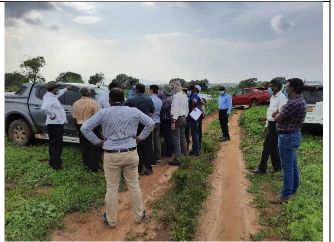
Joint site inspection had participating PUM, PIU and PMDSC-Northern portal-UEC ICB -2A 10 Dec. 2020
