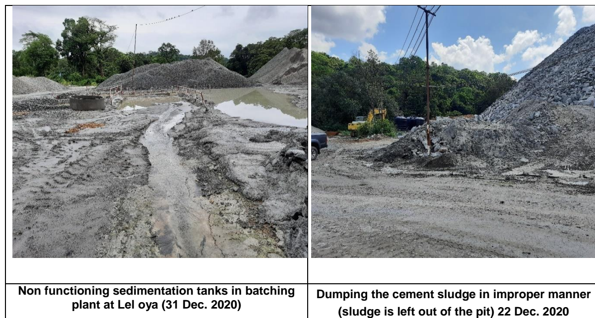
Figure 2-2: Photographic records of Environmental Monitoring in UECP-ICB-2B
