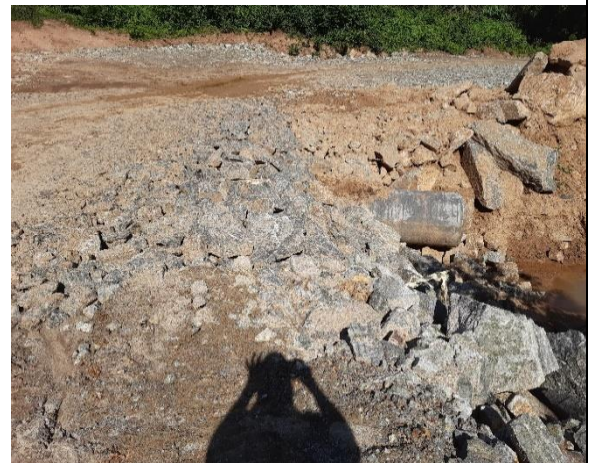
Reinstated providing Hume pipes to manage stream flow (28 Dec. 2020)
