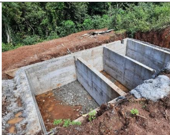
Incompleted sedimentation tanks tunnel 1 inlet (16 Dec. 2020)
