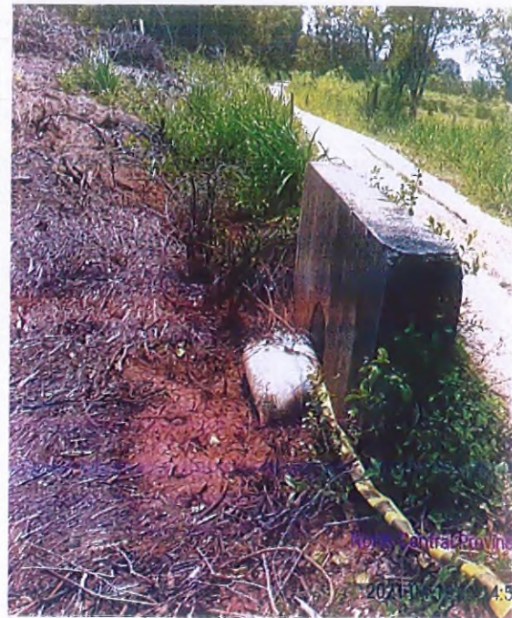
Culvert for the water path.
