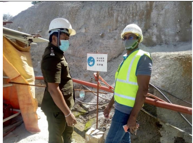
Arranged a site visit by PHI- Lel Oya Tunnel portal area
