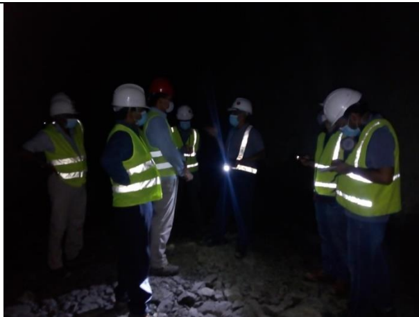
Joint field visit done by PMDSC and Contractor before starting of the works in KMTC
