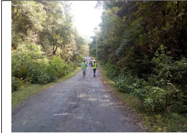
Joint site inspection for utility shifting and tree removal in KMTC Access road
